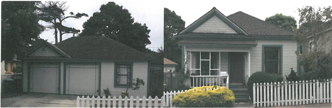
WEST ELEVATION - EXISTING (Composite Photo)
