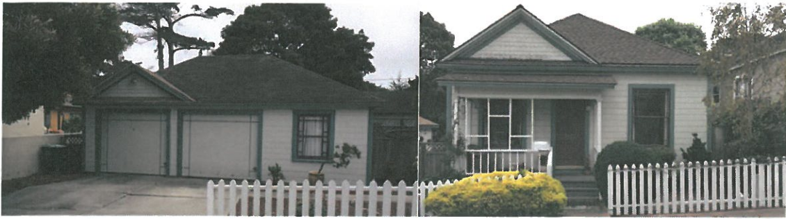
WEST ELEVATION – 213 GRANITE STREET (COMPOSITE PHOTO)
